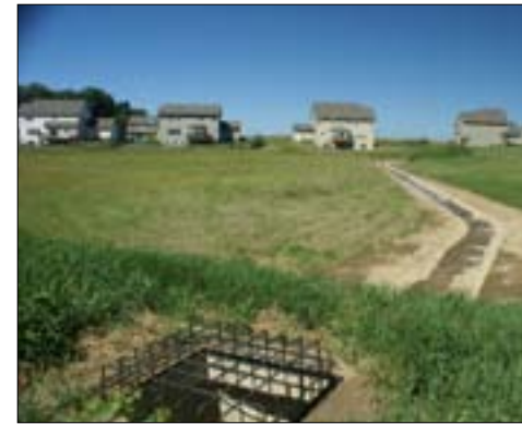
Detention Area with Concrete Channel
