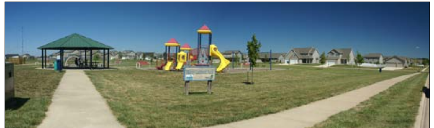
Shelter, 5-12 Play Structure, and Swings (2 belt/2 tot)
