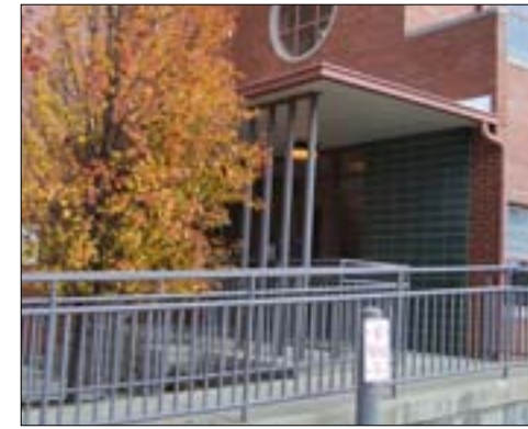
Accessible Southwest Entry
