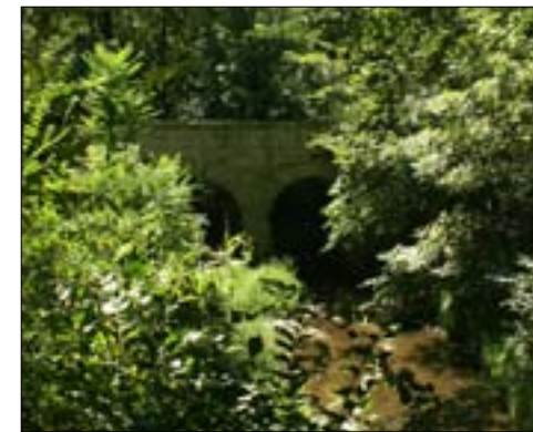
Cemetery Road Bridge - Part of National Historic Registry
